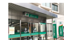
A joint branch that houses Resona Bank's Shijonawate Branch and Kansai Mirai Bank's Shijonawate Branch
